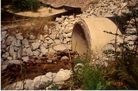
For all exposed crossline pipe ends, when an end treatment is not specified in the plans, use **Pipe Riprap Protection** (804-3xx-xx). For flexible pipe larger than 24" diameter, install pipe straight headwall, pipe end structure, flared end section, or wingwall section in addition to riprap. For all exposed driveway pipe ends where no end treatment is specified in the plans, use **Pipe Riprap Protection** (804-3xx-xx) unless directed otherwise by the engineer.
